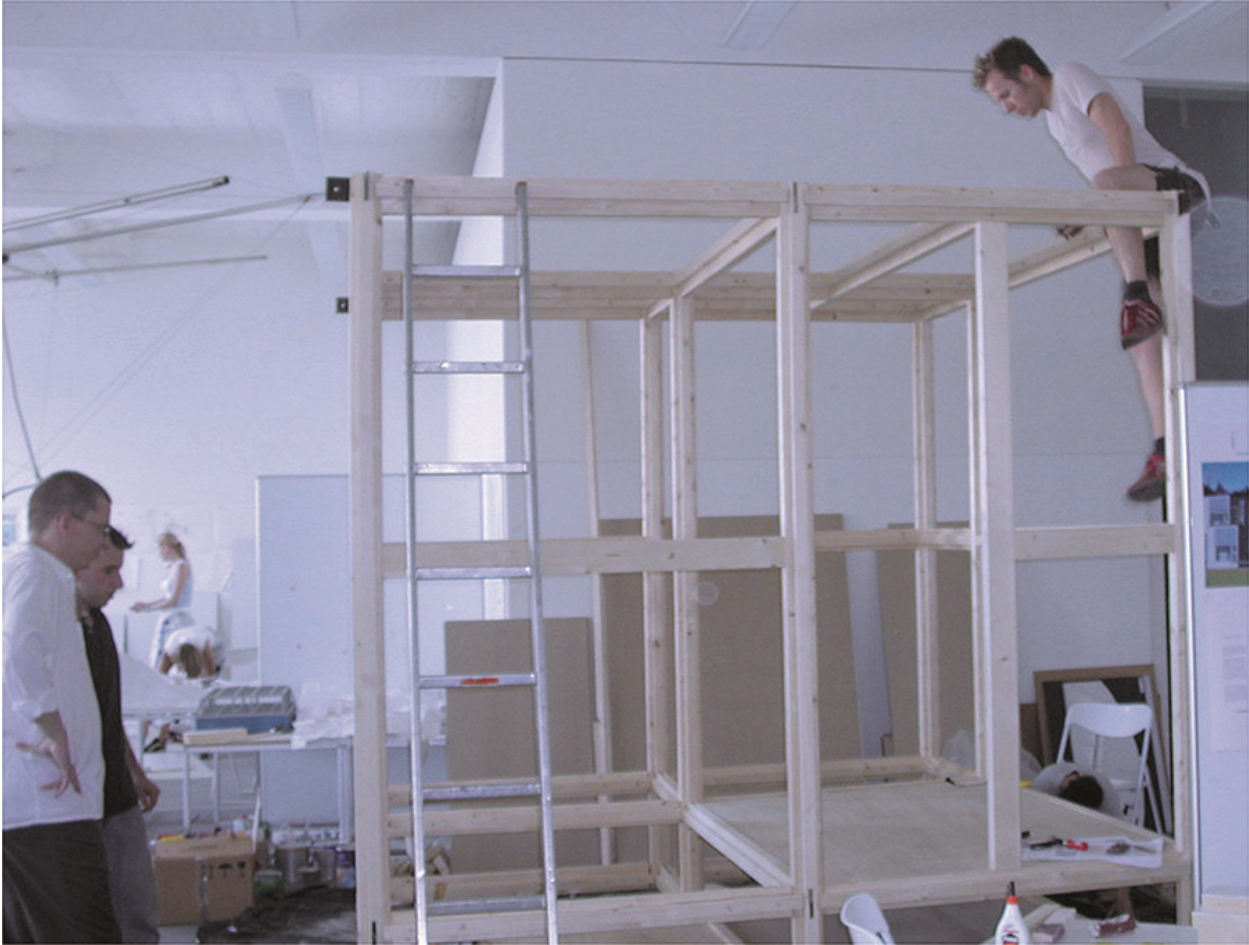
The construction starts with putting the frames together.
